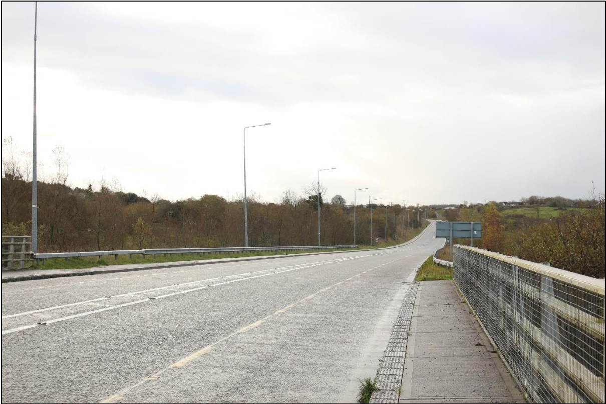
View 09 –Existing - View south from N85 at Claureen River Bridge
