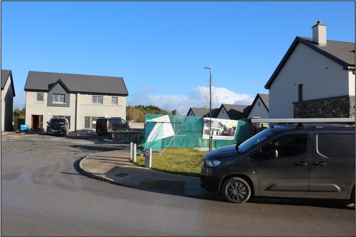
View 5 – Existing – View Northeast from Ballymacaula View
